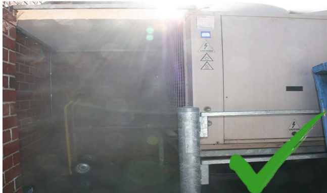
An OzMist Pre-Cooling system flash evaporates the hot air particles leaving no wet surfaces, while effectively reducing the ambient air temperature around the condenser units.
