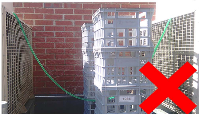
Traditional sprinkler setups around condenser units can cause corrosion on the fins and lead to excessive water use. Excess water can also lead to potential OH&S issues by leaving wet surfaces around the units.
