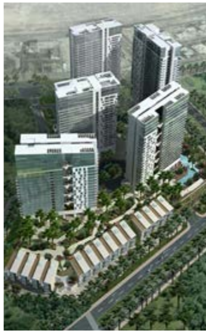
Chilled Water Plantroom Design & Commissioning Evaluation for 5 towers (Rihan Height, Abu Dhabi) The project consists of 5 Chilled Water Plantroom requiring Design and Testing and Commissioning Evaluation.
