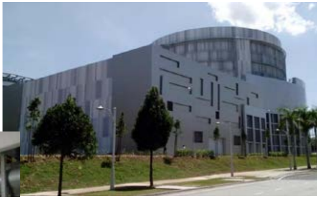
GDC Chilled Water Thermal Energy Storage Plant, Putrajaya
