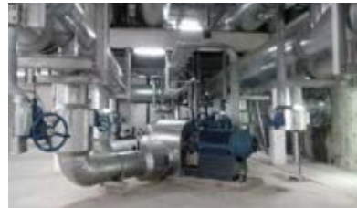
The project is as 100,000 RThr, Chilled Water Thermal Energy Storage Tank, Plant and pump station. The system was designed to cater for tie in with future extension without disruption to the operation.
